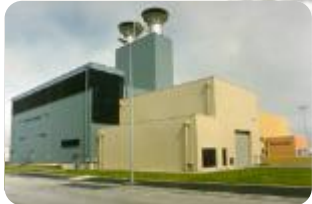
Areva - La Hague facilities
